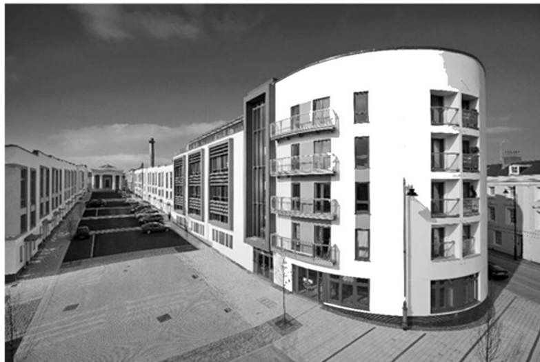
Figure 5: Examples of new buildings in conservation areas making a positive contribution to setting
