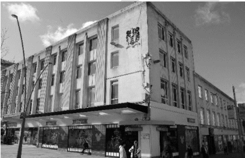
Figure 19: The formal style of this building reflects its status as an important corner of the Abercrombie plan for Plymouth
