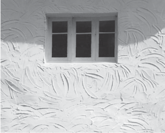
Figure 15: Renewing the render of this cottage was appropriate, but not the added patterning
