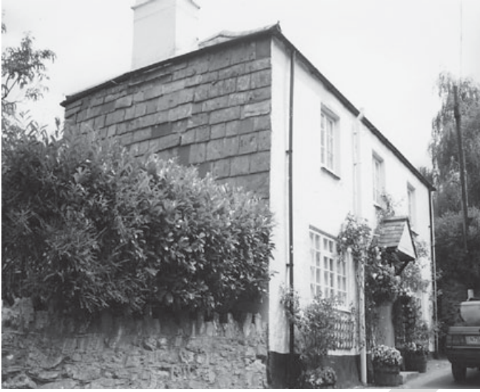
Figure 13: This prominent slate cladding is attractive, but its use can be rare and needs to remain so to preserve its particular identity
