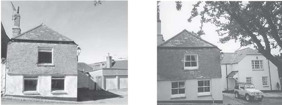
Figure 11: Before (left) and after (right) example of redevelopment where siting was a key consideration
