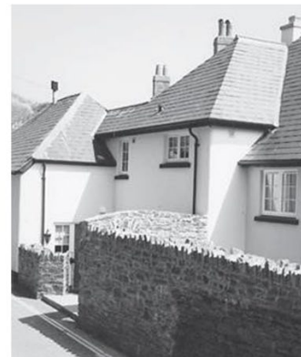
Figure 21: This small development is modern, but it is suited to its village setting, both in terms of its overall vernacular styling as well as the quality and subtle detailing of its parts. Note, for example, the softened corners to the rendered walls and the appearance of the roof with its traditional 'mitred' hips (right) in comparison to the existing tiled ones (left).
