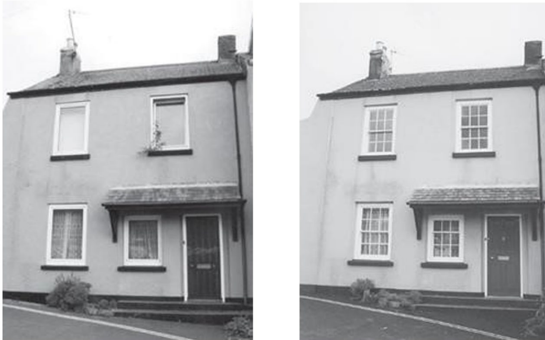
Figure 1: Before (left) and after (right) restoration
