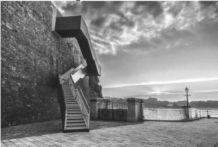
Figure 20: The new staircase linking the Royal William Yard to Devils Point successfully introduced a distinctly modern architectural style and materials to the historic victualling yard. Image © Jay Stone
